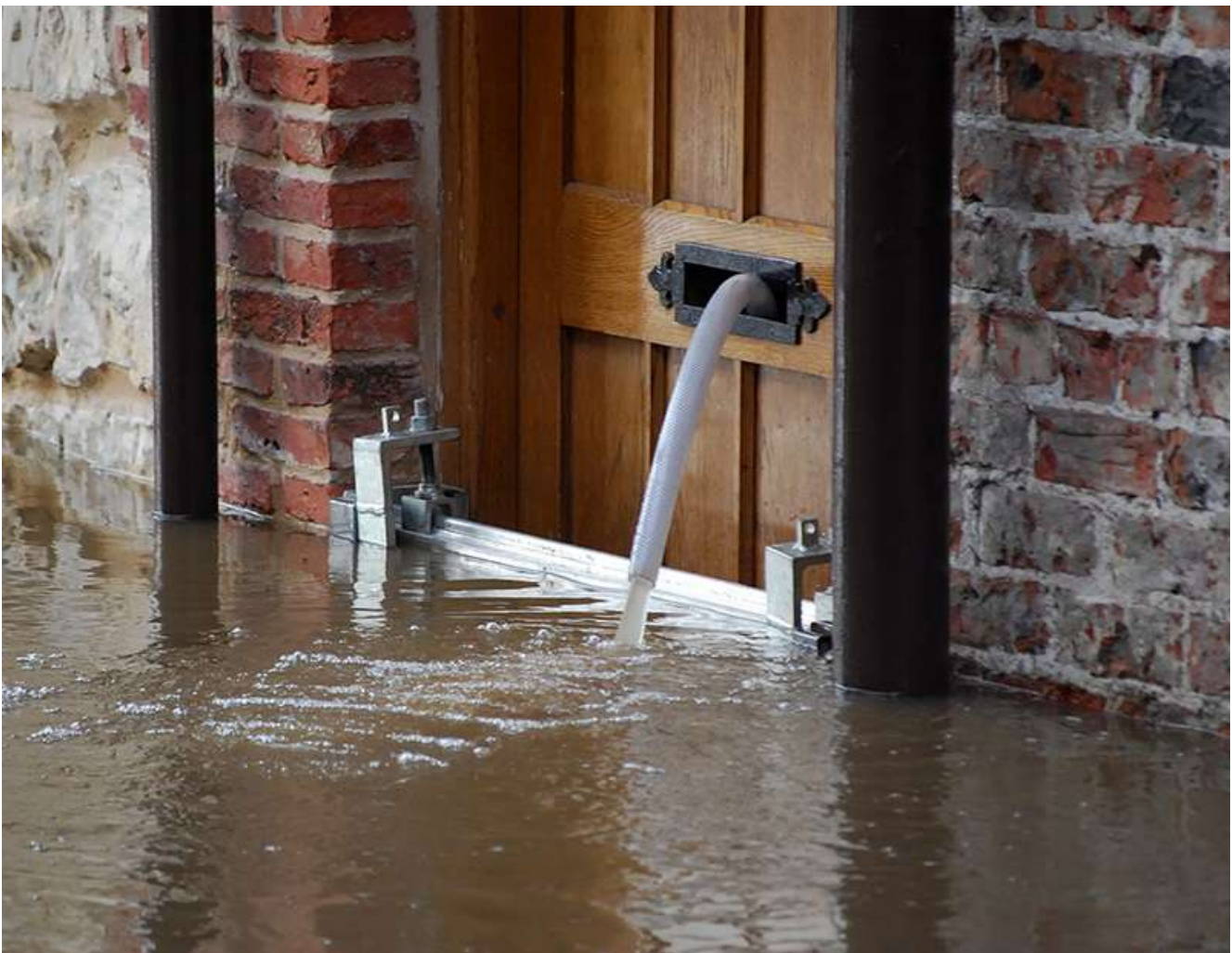
Floodwater being pumped from a property in Gloucester.
